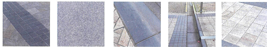
Semi-mountable Kerb Black oxide to match existing Chapel St Plaza works
