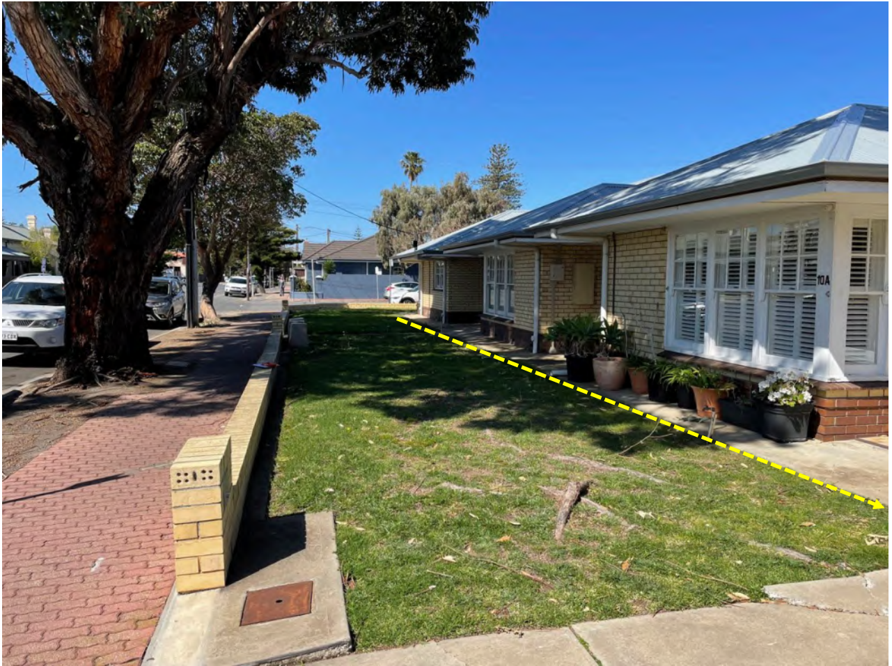
Figure 2. The subject site and tree, looking approximately east along the front yard of 10A Augusta Street on the 23 rd of September 2021. The superimposed yellow line indicates the proposed alignment of the root barrier as outlined by Ben Hall of the City of Holdfast Bay). Note the presence of numerous surface roots in the front lawn yard of 10A Augusta Street.
