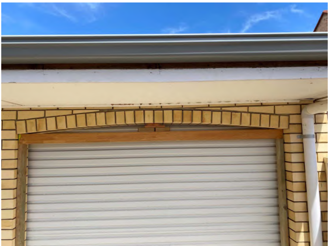
P11 Garage arch – showing timber framing to sides and top
