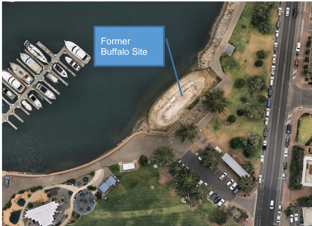
Figure 1- Aerial view of the site, from Nearmap.
