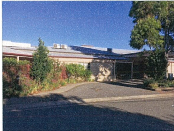
Existing aged care accommodation
