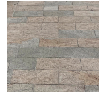
Feature Paving + Crossovers Feature Paving: Urbanstone Juperana Granite - 400 mm x 200 mm in Stretcherbond with inlay
