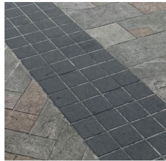
Feature Paving + Cobbleset Paving Bands Footpath Banding: Austral Black Stone-100 mm x 100 mm (charcoal oxide mortar)
