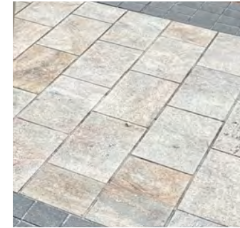
Footpath, Feature + Crossover Paving: Juperana Granite
