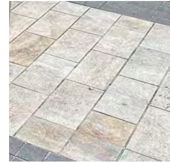
Footpath, Feature + Crossover Paving: Juperana Granite
