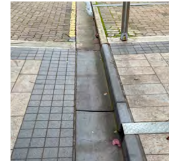
Upright Kerb Black oxide to match existing Chapel St Plaza works
