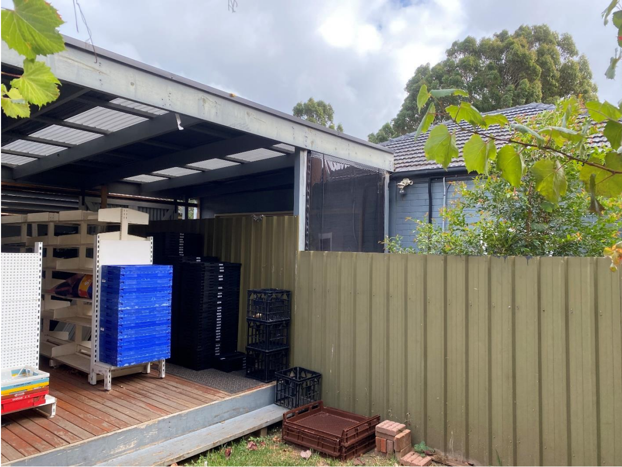
Above: View north showing the location of the fence between the grocery and the existing dwelling
