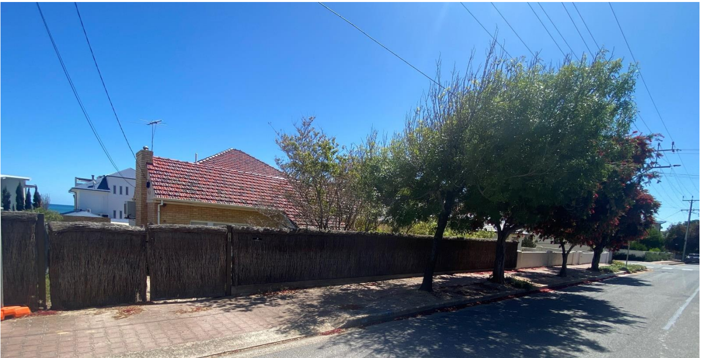
Figure 2: Streetscape image of the subject site
