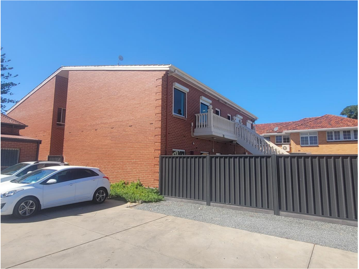
Photo showing the neighbouring property to the south
