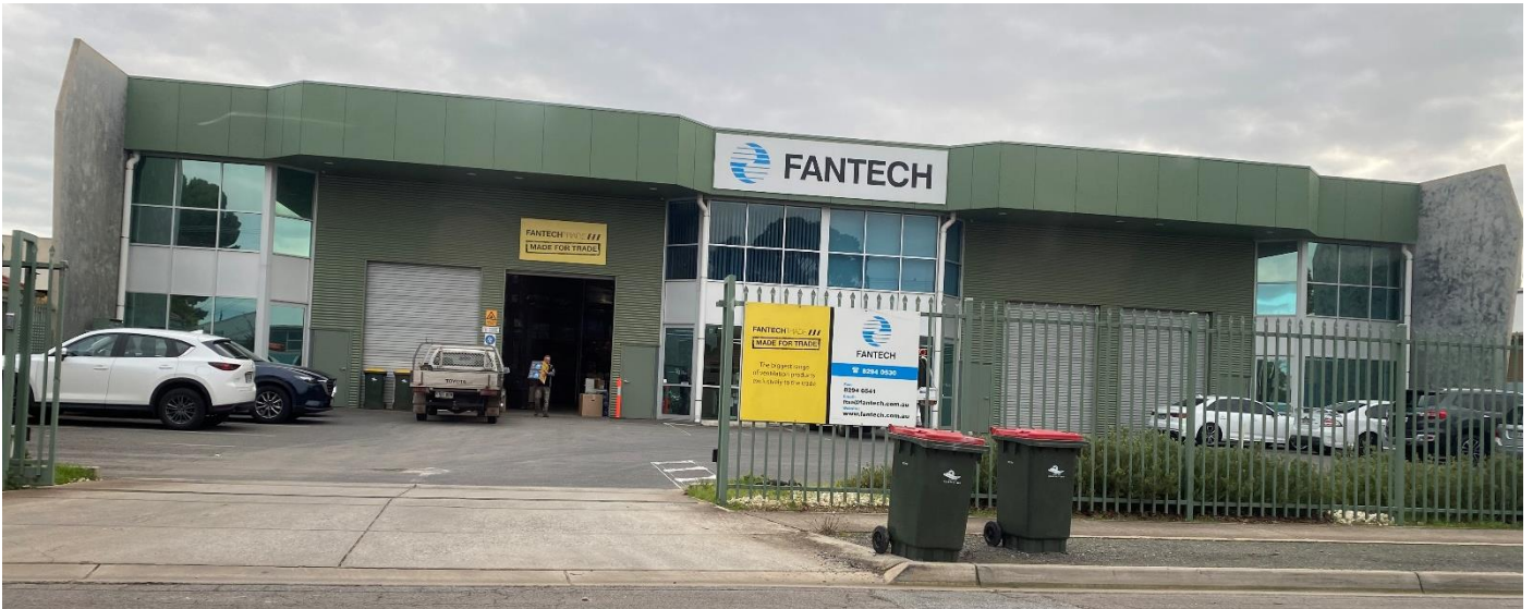
Below: 52 to 54 Paringa Avenue
