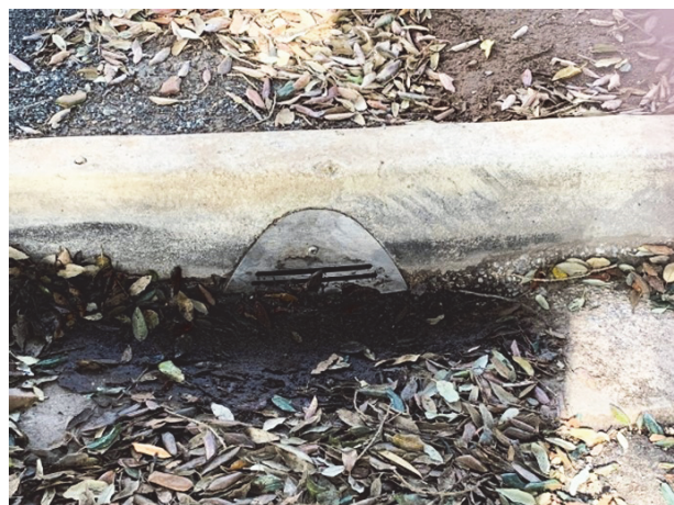
Figure 5.5: Examples of WSUD under Norfolk Pines in Glenelg and a street tree inlet to redirect stormwater to tree roots in South Brighton
