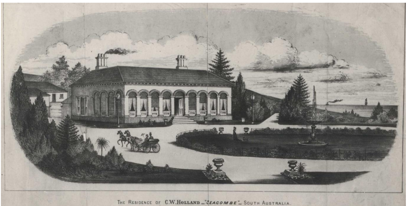
Seacombe House Circa 1880, Holdfast Bay History Centre PH-AH-03128
